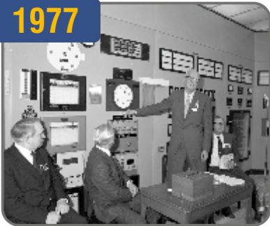
Experimental Fast Reactor shut down
