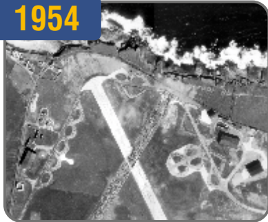
UK Government selects wartime airfield at Dounreay as site for fast reactor research and development
