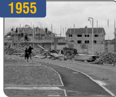
UKAEA starts building housing estate in Thurso
