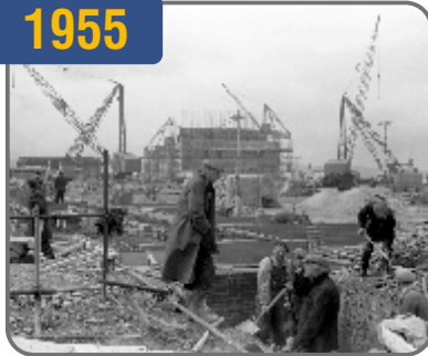
UK Atomic Energy Authority begins construction
