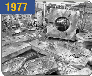
Explosion in underground waste shaft
